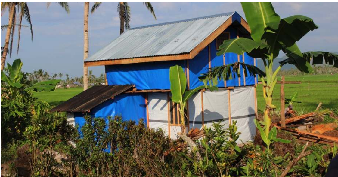
A shelter kit with temporary tarp walls
