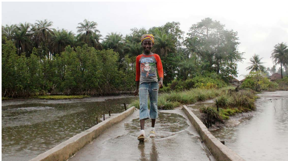
Ellen crosses the new bridge built with ActionAid's support. PHOTO: JONATHAN BUNDU/ACTIONAID
